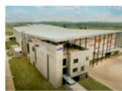
Tajlandia Chonburi LGH CRANES CO., LTD. T: +66 (0)-2327 9399 ghthailand@ghcranes.com
