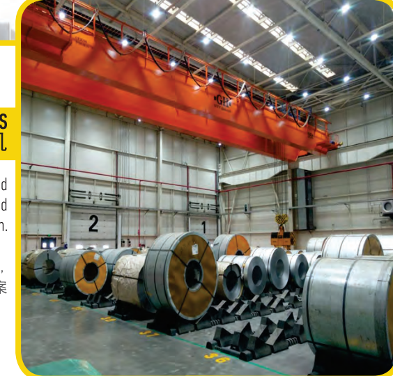
COIL WAREHOUSE MANAGING CRANES 钢卷仓库起重机
