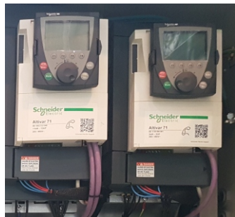
11 / Trolley Frequency inverter
